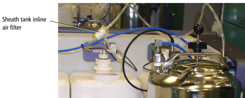
Figure 6-18 Inline air filter for sheath tank
